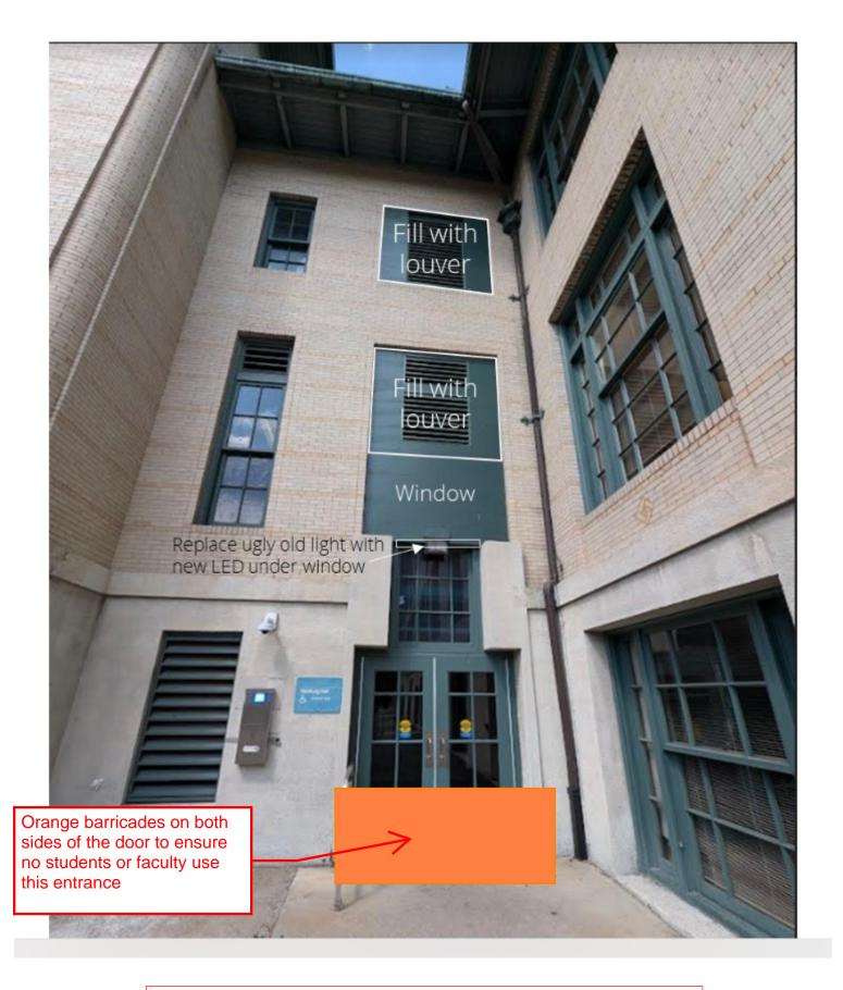
Workers will be doing the install via a scissor lift where they will be tied off to ensure they are protected from fall hazards. Inside the building the wall beneath the window is not adequate height so we will be tying off to a safe load capable structure. An additional employee will be monitoring the area to ensure nobody enters during lifting.
